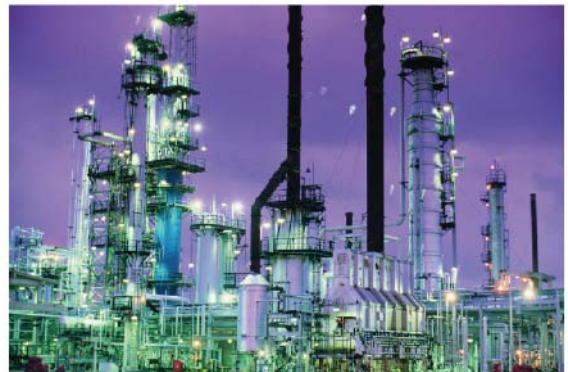
Solutions for Oil & Gas Downstream
